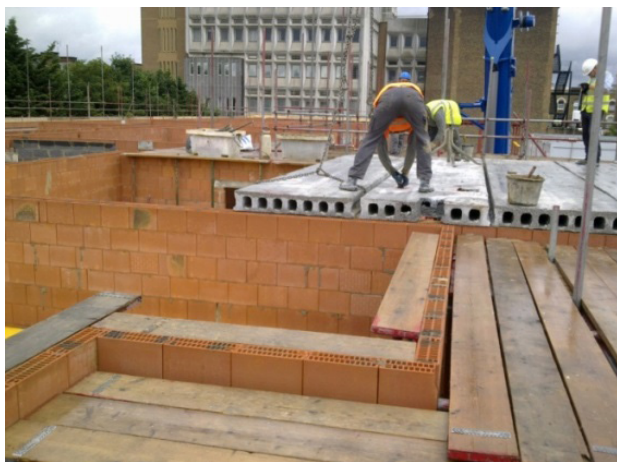
Planks being located close to final position using choke chains.
