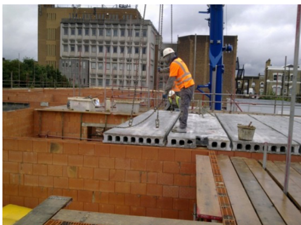
Final positioning utilising lifting eyes.
